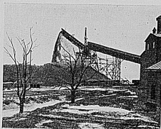
THE RESIDUE OF SAND, AFTER SEPARATION FROM THE IRON, BEING DEPOSITED IN A HEAP.
